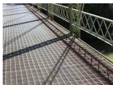
Steel grating bridge decks
