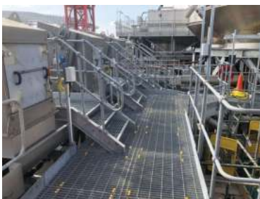
Steel grating platform mezzanine
