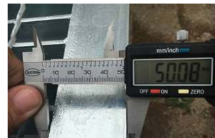
Angle bar size inspection
