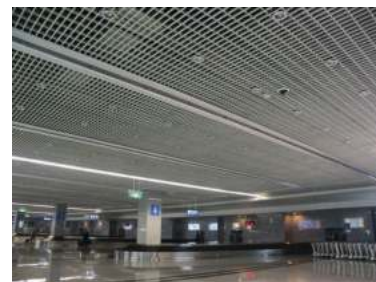
Steel grating ceiling
