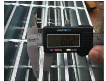
Bearing bar size inspection
